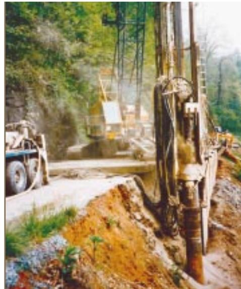
DR-24 mast kit mounted on crane leads to set foundation pilings for a retaining wall.
