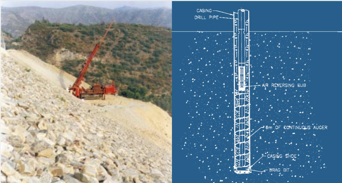
Foremost DR-24 working at dam site. Because of concern over blowout potential, an air-reversing sub was positioned 6m (18ft) above the drill bit to divert air flow back up the annulus to clear cuttings from the auger string. The tooling configuration created a low-pressure vacuum at the bit, eliminating the possibility of a blowout.
